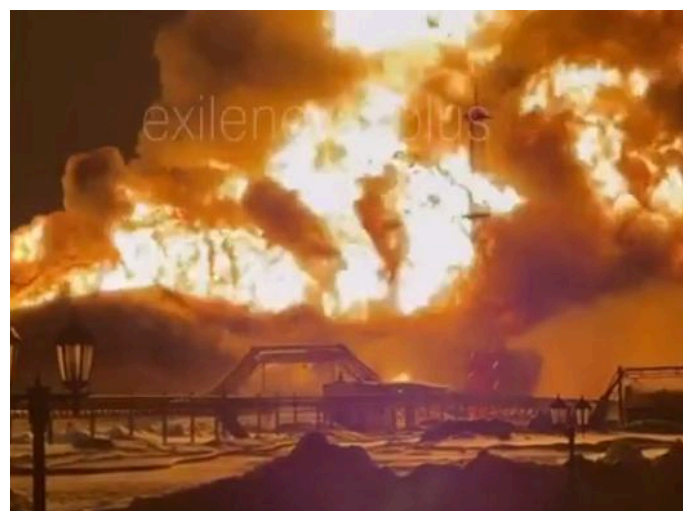
Massive Fire After Attack on Kaleykino Oil Pumping Station.
