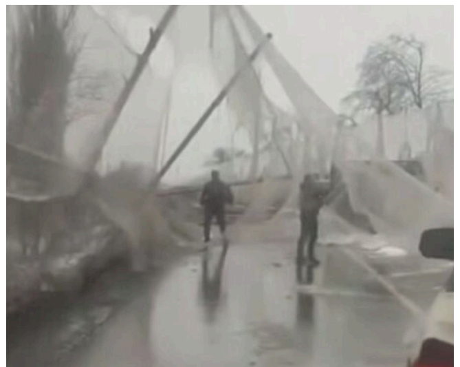
Collapsed Anti-Drone Nets. Source: pekhno_news
