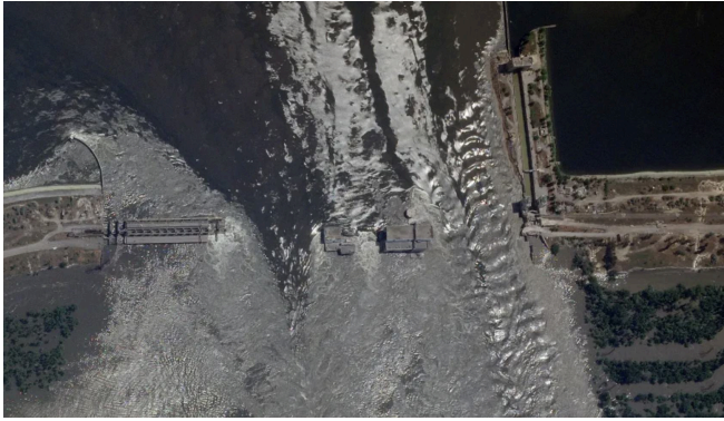
Destroyed Khakovska Dam, Kherson region, Ukraine 2023. Source: TWZ
