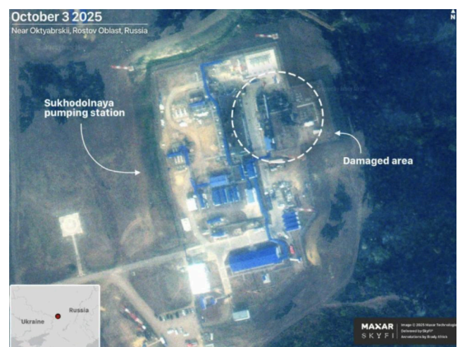
Sukhodolnaya oil pumping station. Source: Maxar .
