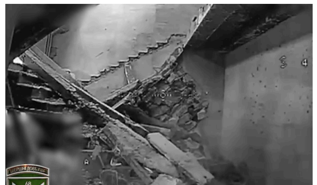
Fiber-Optic Drones inside destroyed apartment building. Source: Shershni Dovbusha
