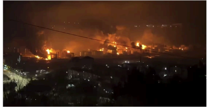
Fire at Tuapse Oil Refinery Following the April 20 Strike. Source: exilenova_plus
