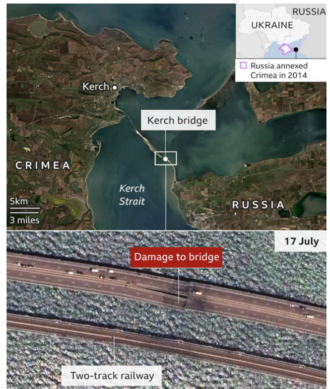
BBC. Satellite footage of the damage to the Crimean Bridge. 55
